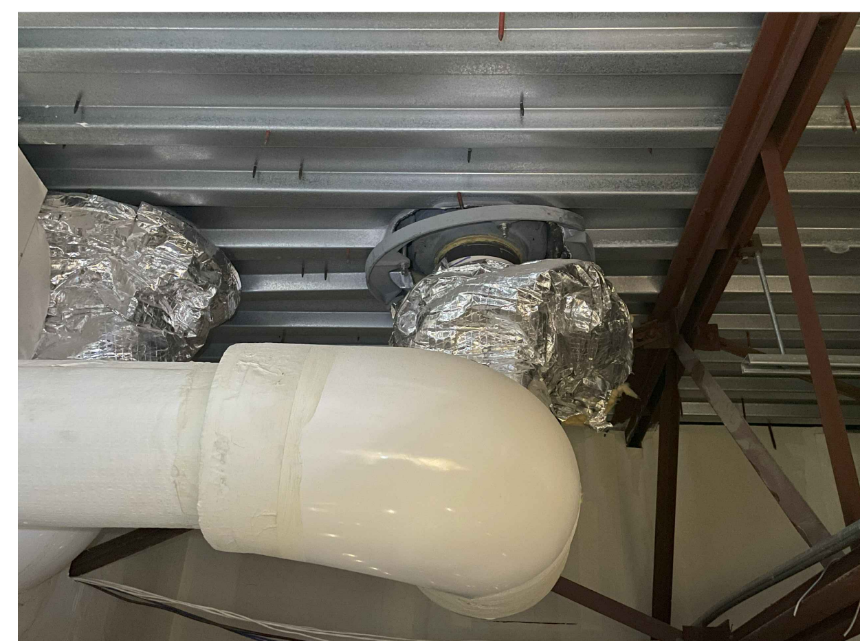
Roof Drain Penetration * Remove roof drain assembly. * Verify integrity of modified bitumen roofing membrane at roof drains. * Reseal penetrations and apply roof sealant. * Install new roof drain and overflow assembly. * Clean and water test the drain lines from the roof thru the discharge point.
