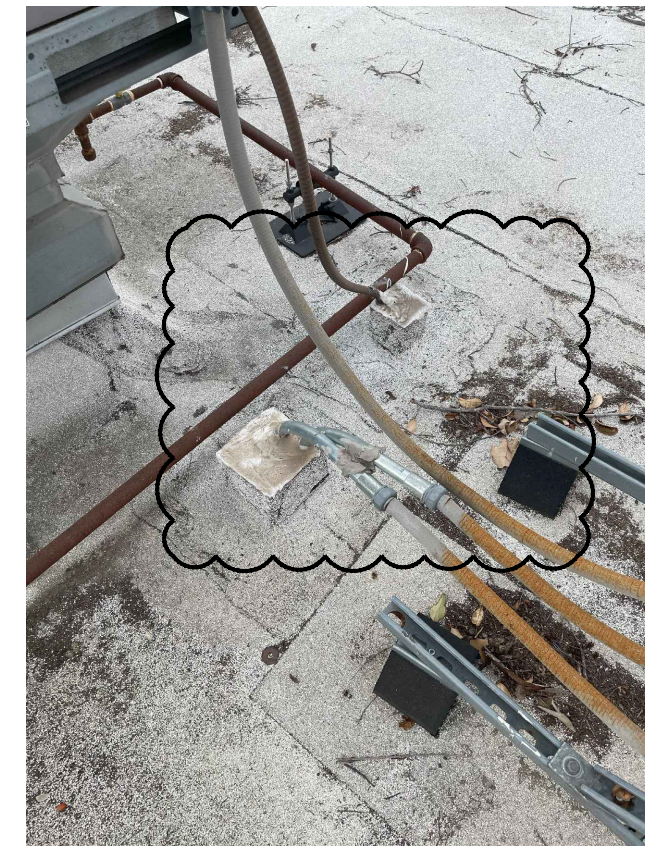
Electrical Roof Penetration * Remove sealant and mastic at conduit and unistrut roof penetration. * Verify integrity of modified bitumen roofing membrane at penetration curb. * Reseal penetrations and apply roof sealant. * Install new weatherseal, cover and gasket at electrical outlet and j-box. Refer to 02/A2.05, 03/A2.05.
