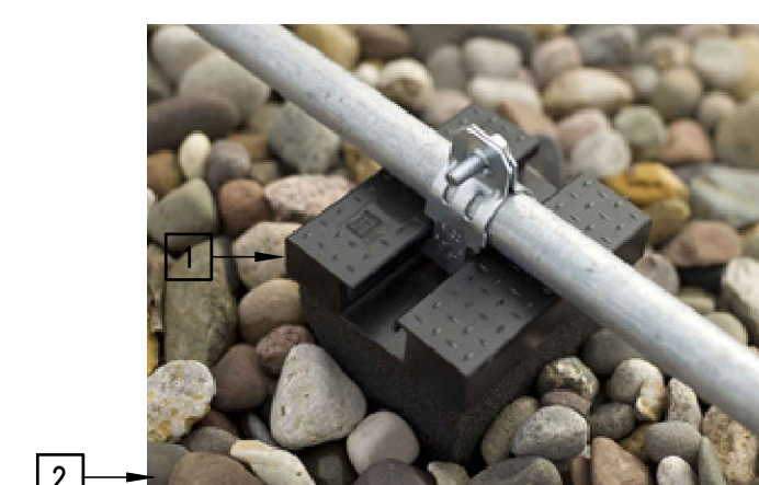
15 ROOF MOUNTED RACEWAYS SUPPORT DETAIL SCALE : NOT TO SCALE
